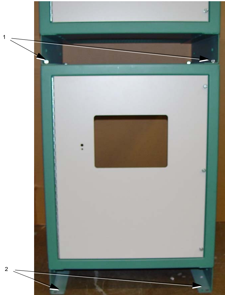
Figure 12: Location of Bolts for Stacking CCRs
