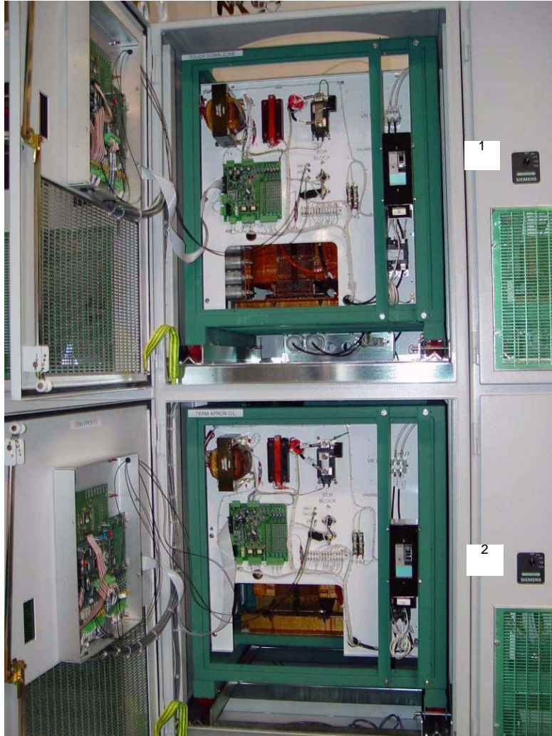
Figure 14: Powerpack Installation in SGRS
